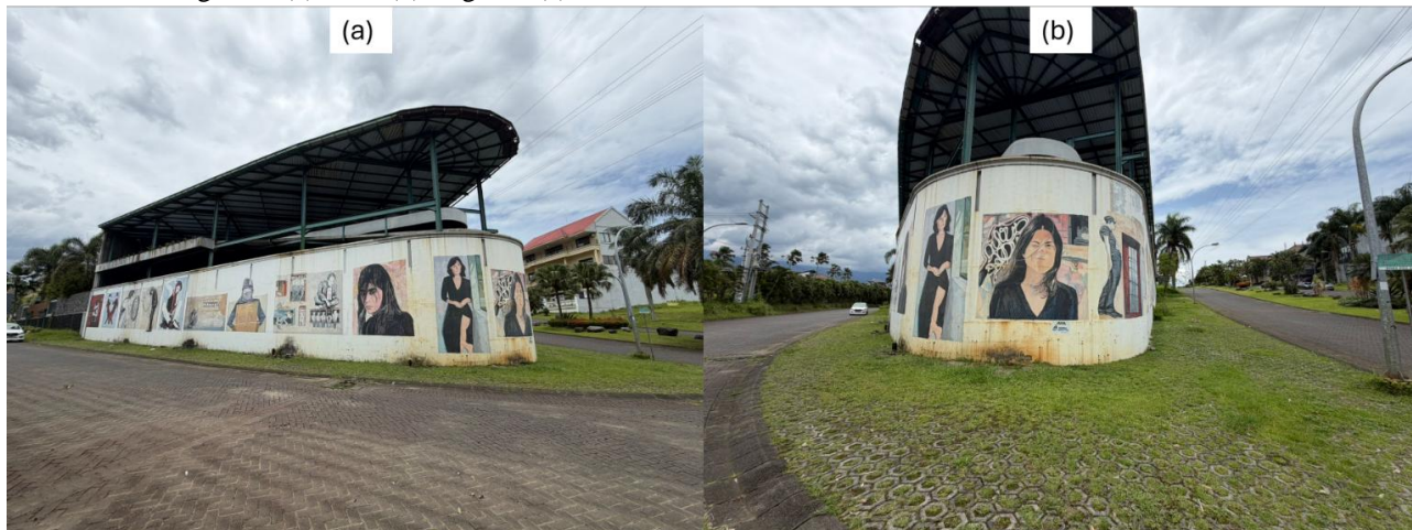
Figure 1. (a) field photo of the mural main facade; (b) field photo of the curved facade
